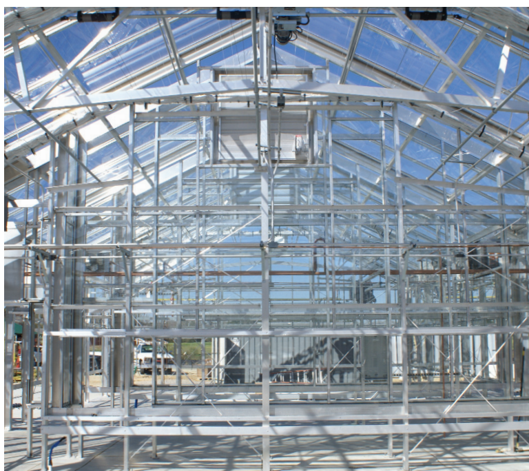
FIGURE 9. Aluminum Framing*
