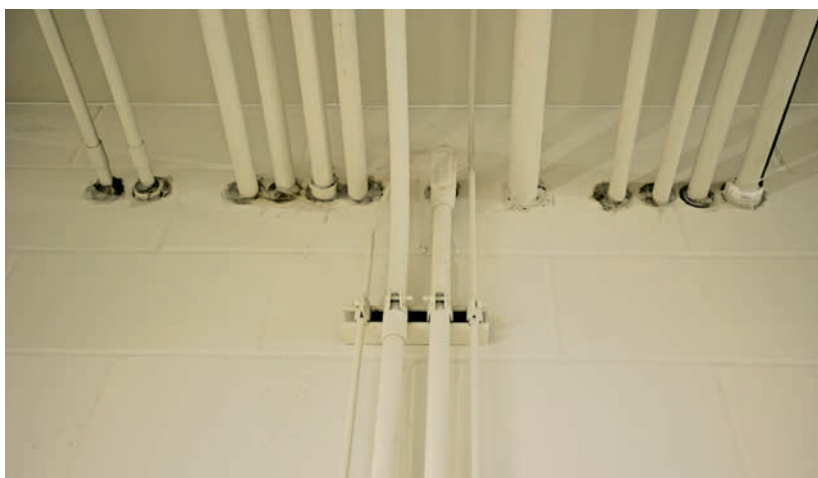
FIGURE 18. Caulking around Service Intrusions*
